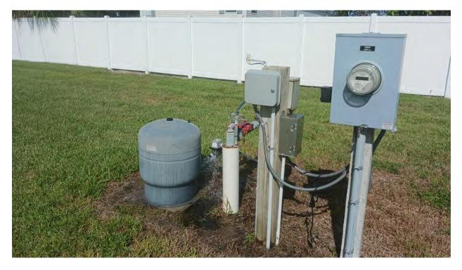
Pressure relief valve is blown as a result of the pump coming on due to a faulty pressure switch. The pressure gauge, pressure switch and pressure relief valve were all replaced and are working properly.
